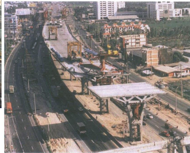
Fig. 18. Overview of progress in erection of bridge superstructure.
